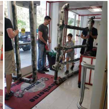
Time was also spent dismantling and removing our aquaponics system. Unfortunately, the system needed too many repairs.
