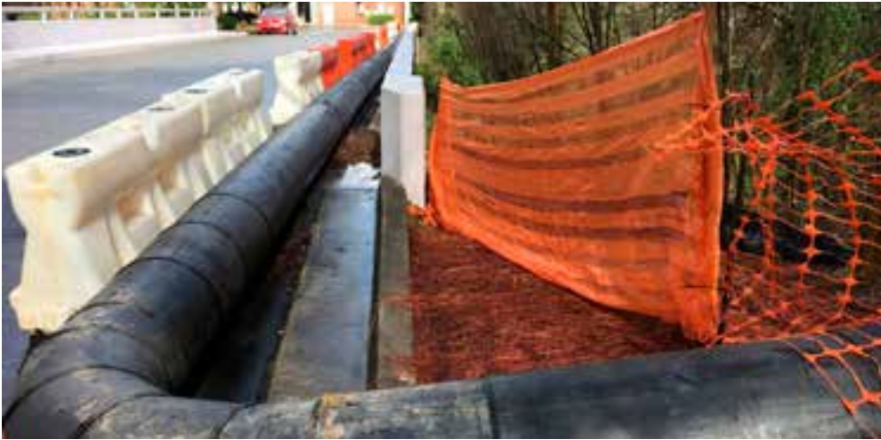
This shows the new sewer pipe before it was buried. In the photo, the pipe is stretched across the Flowers Road bridge over the North Fork.
